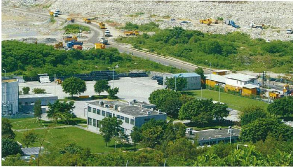
Site office area of SENT Landfill
